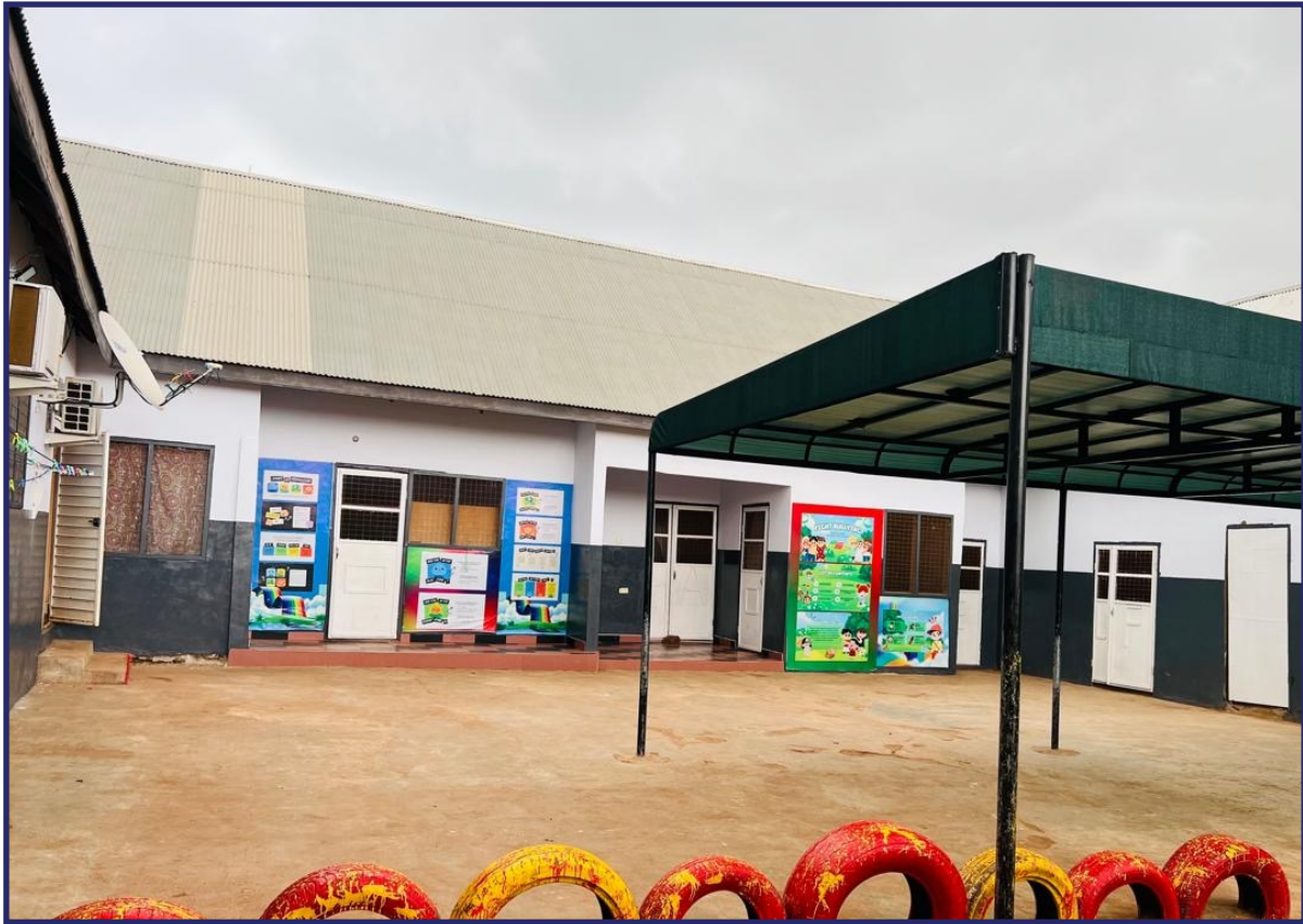
Figure 8: Daycare centre at the Assistance Hub, Tamale
